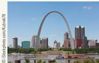
The Gateway Arch in St. Louis, Missouri, is shaped in the form of the graph of a combination of exponential functions ( not a parabola, as it might first appear). Specifically, it is a catenary , which is the graph of an equation of the form
